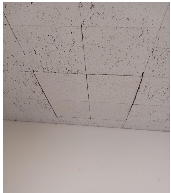
Northern Branch Courthouse – Fire Protection
