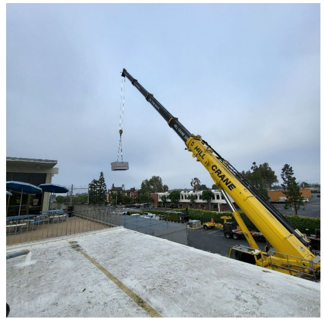
West Justice Center – HVAC (BMS)
