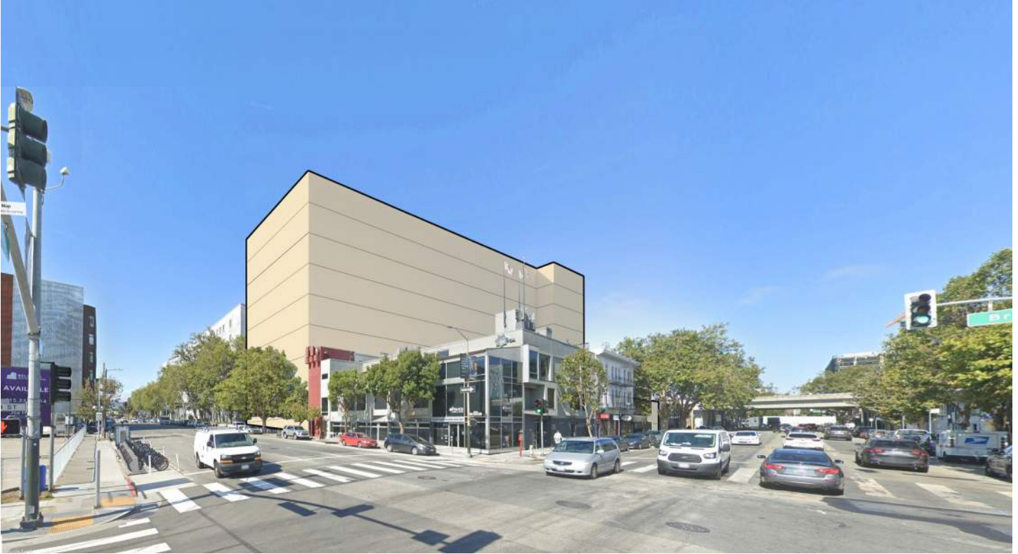
VIEW FROM INTERSECTION OF BRYANT STREET AND 6TH STREET WITH (E) HALL OF JUSTICE
