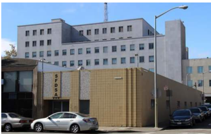
Figure 3. 444 6th Street – built 1959.
