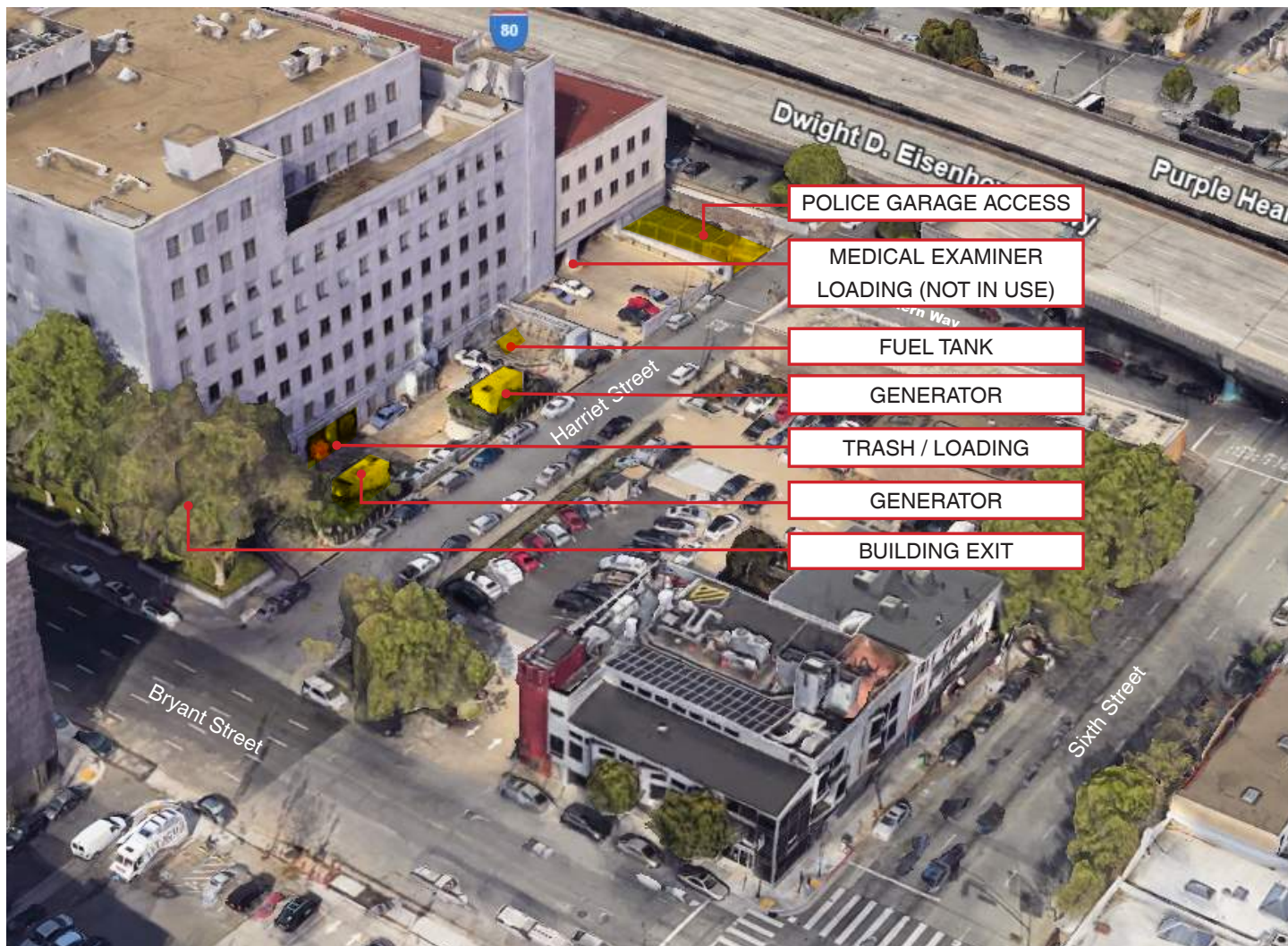
Aerial of existing Hall of Justice Loading Area
