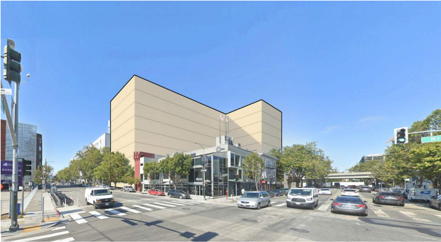
VIEW FROM INTERSECTION OF BRYANT STREET AND 6TH STREET WITH (E) HALL OF JUSTICE
