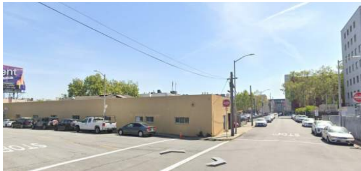
Street view from Ahern Way looking south at Harriet Street
