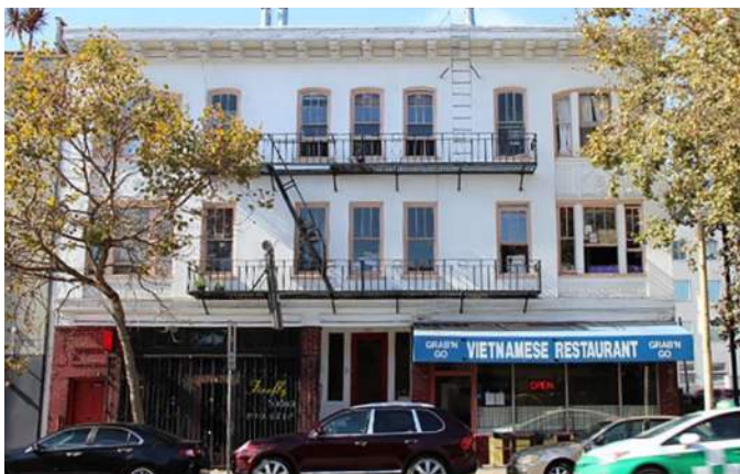
Figure 5. 480-84 6th Street – built 1916.
