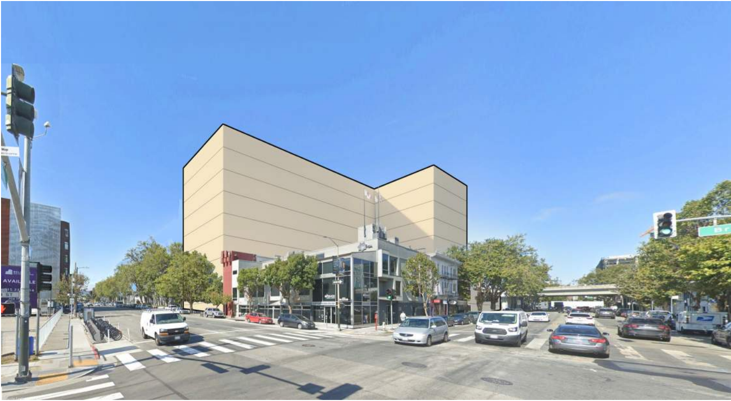
VIEW FROM INTERSECTION OF BRYANT STREET AND 6TH STREET WITHOUT (E) HALL OF JUSTICE
