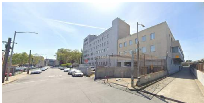
Street view from Ahern Way looking south at Harriet Street
