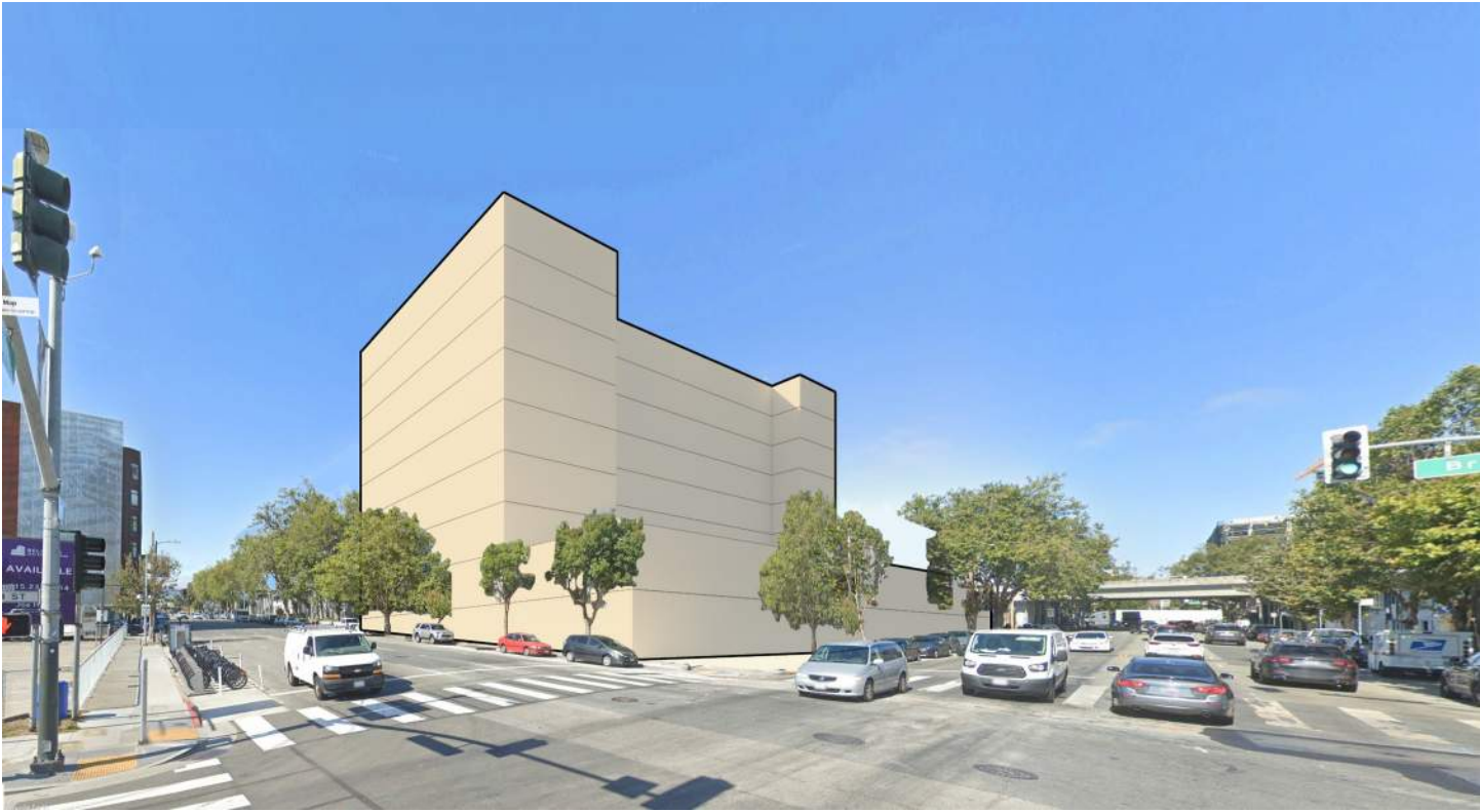
VIEW FROM INTERSECTION OF BRYANT STREET AND 6TH STREET WITHOUT (E) HALL OF JUSTICE
