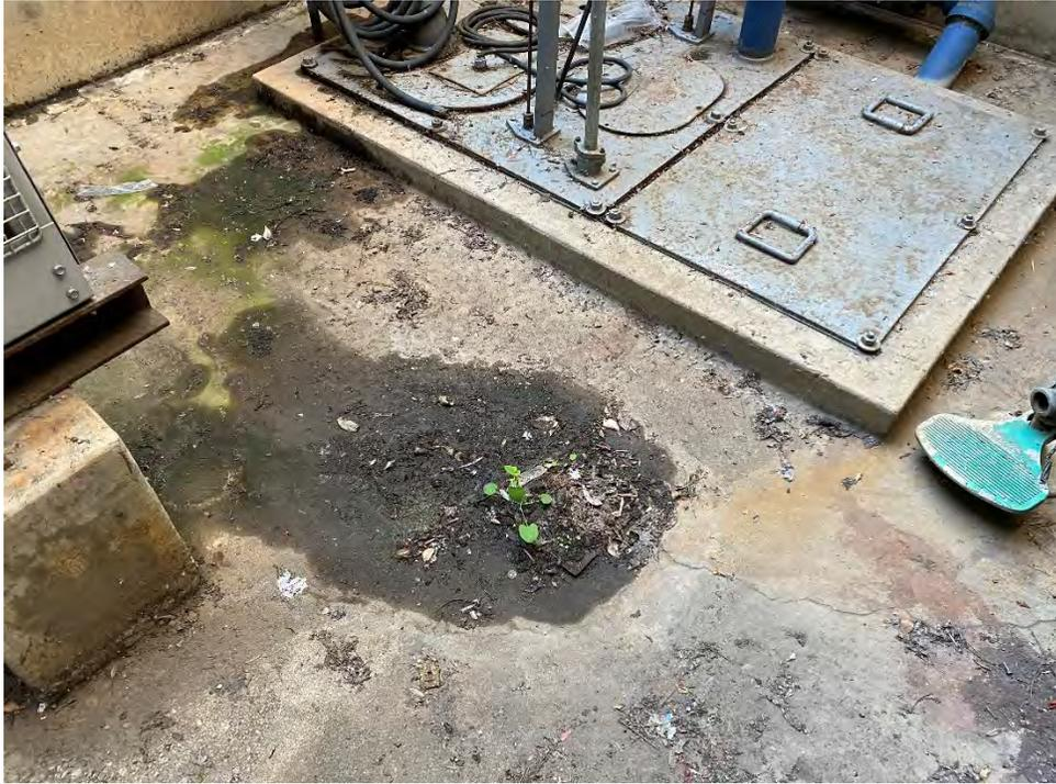
**Photo #13** View of floor drain in the center of the outdoor basement area. The rusted grate is clogged with soil and plant debris and staining is visible around the grate.
