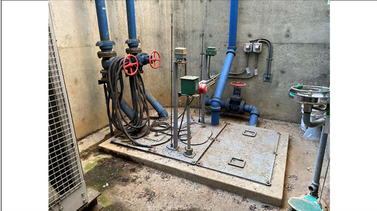
**Photo #9** View (looking southwest) of the underground sewage pump located in the outdoor basement-level area located south of the basement electrical and mechanical rooms. This sub-grade area is covered at street level with a metal grate located west of the main entrance to the building. Note evidence of surface staining.
