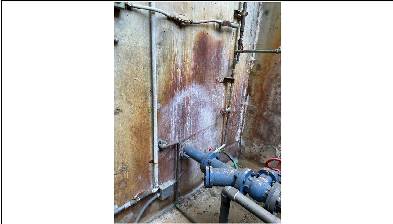
**Photo #12** Alternate view (facing northeast) of staining on the northern cement wall of the outdoor basement area adjacent to the cooling tower.
