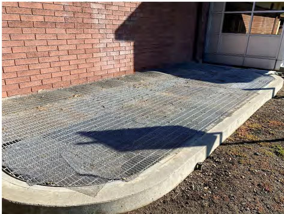
**Photo #20** View (facing northeast) of the metal grate covering the outdoor sub-grade basement area which houses the cooling tower and sewer pump. The windows in the top right of the photo lead to the main entrance area.
