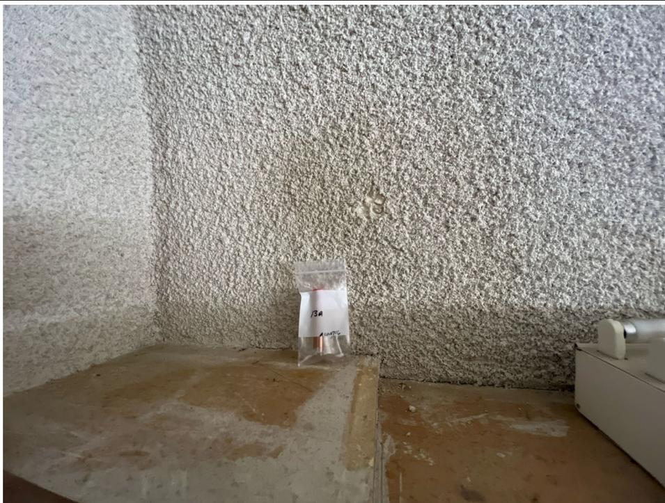
**Photo #4** View of white acoustic ceiling texture (HA #13). This material is asbestos-containing.
