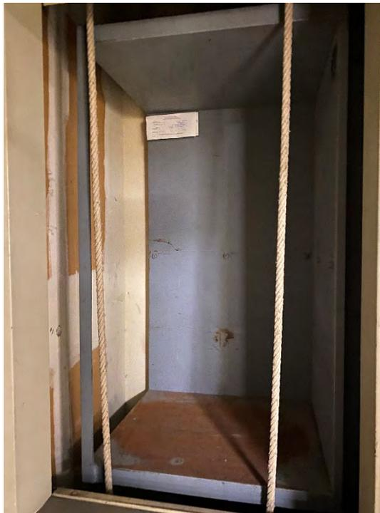
**Photo #2** View of dumbwaiter located in the southwest corner of Subject Property building. The dumbwaiter appears to be controlled manually by ropes and contains no hydraulics.
