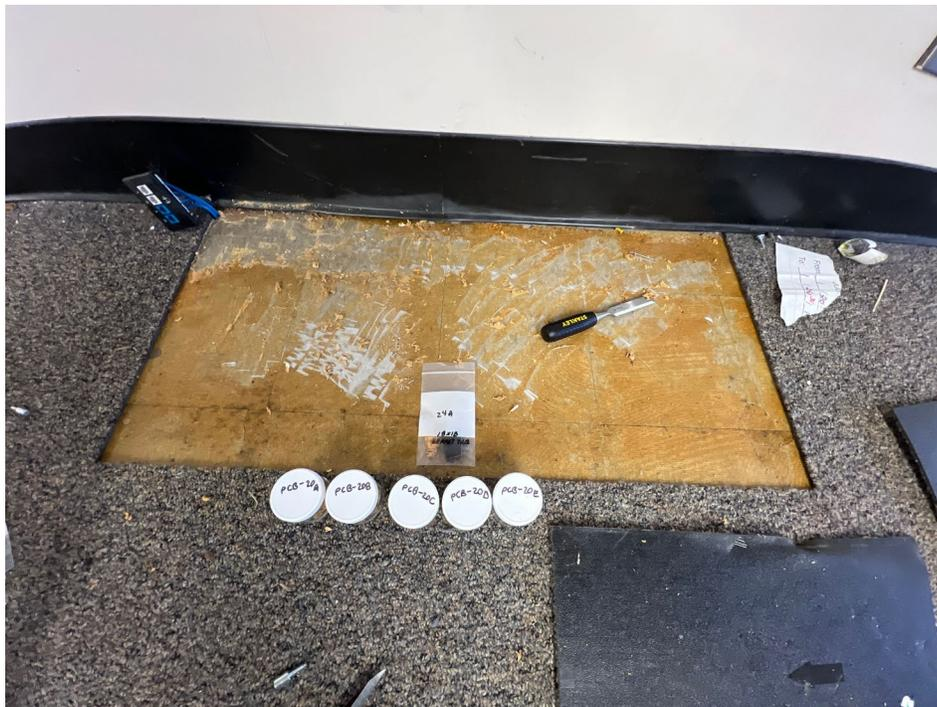
**Photo #8** View of gray/tan/orange carpet adhesive (HA #24) associated with carpet tiles. This material is asbestos-containing.
