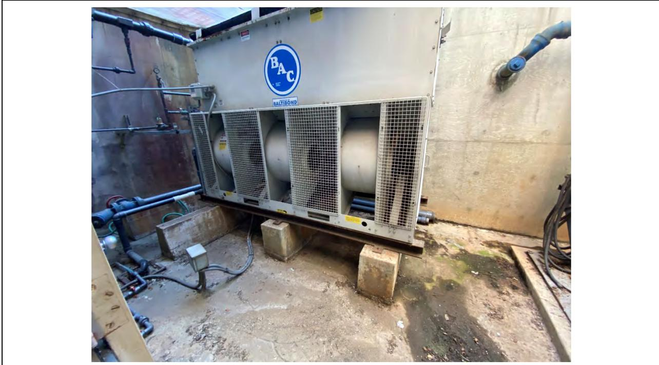
**Photo #11** View (facing southeast) of the cooling tower which is also housed in the outdoor basement area. The eastern cement wall of the area (visible at left of frame) is heavily stained and surface staining was also noted adjacent to the cooling tower and sewage pump (right of frame).
