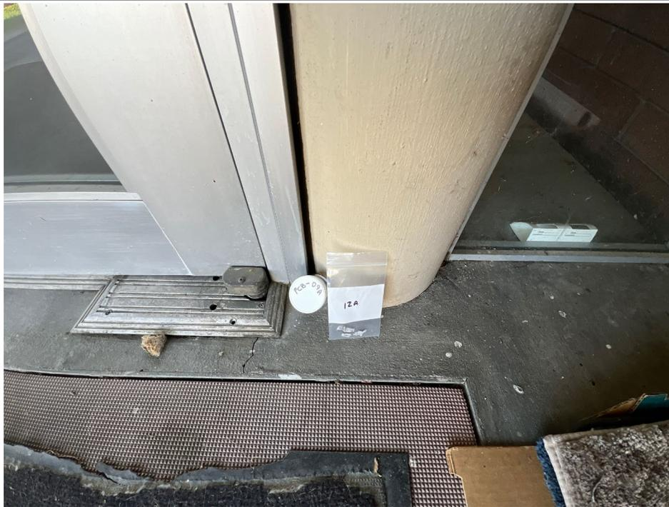
**Photo #3** View of gray window putty associated with exterior windows (HA #12). This material is asbestos-containing.
