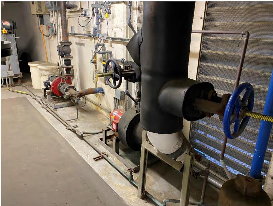
**Photo #4** Alternate view (looking southeast) of basement mechanical room. Note rusted piping and two white poly containers (contents unknown) visible at left of frame.
