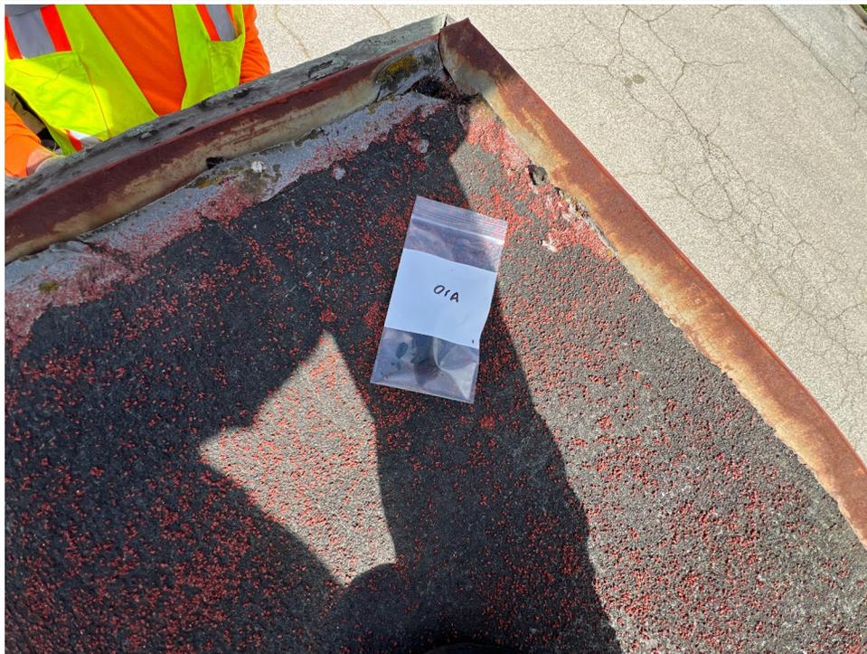
**Photo #10** View of the shed roof system (HA #01 SHED). This material is asbestos-containing. The black roof penetration sealant (HA #02 SHED) is also asbestos-containing.
