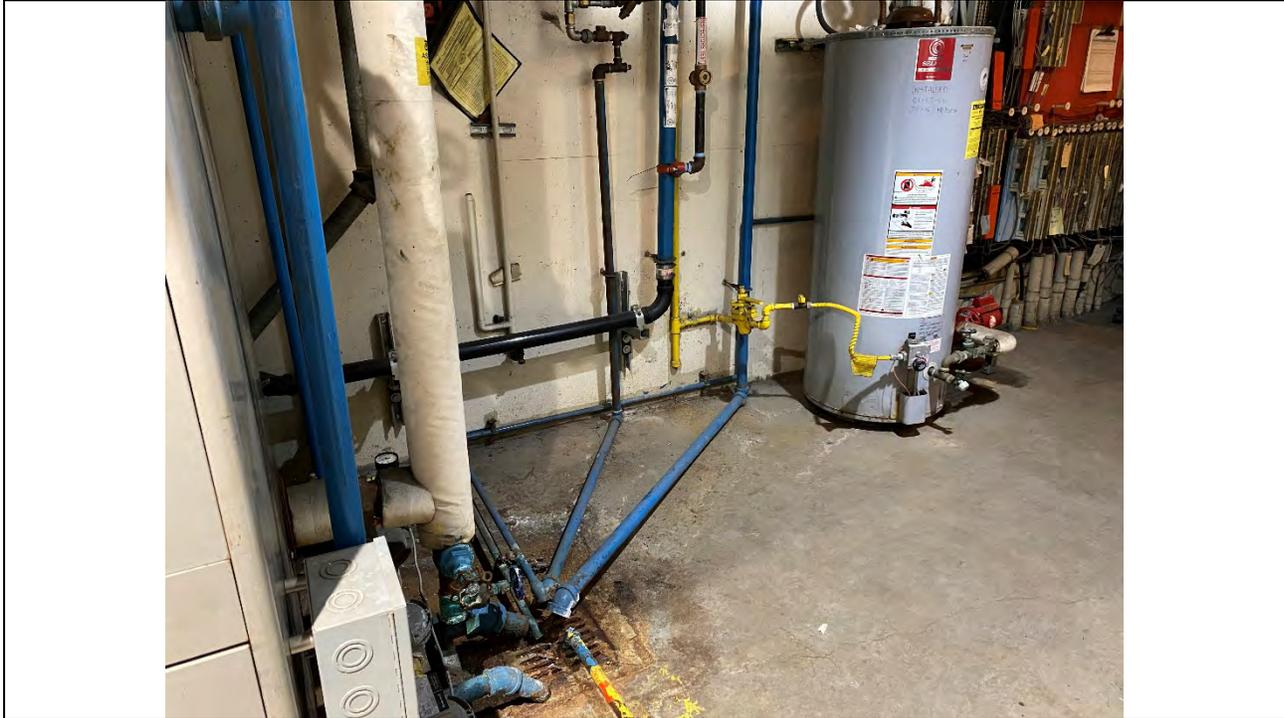
**Photo #5** View (looking southwest) of basement electrical room (located west of the mechanical room) which contains an electrical board and water heater. Note the rusted/corroded floor drain with evidence of staining.
