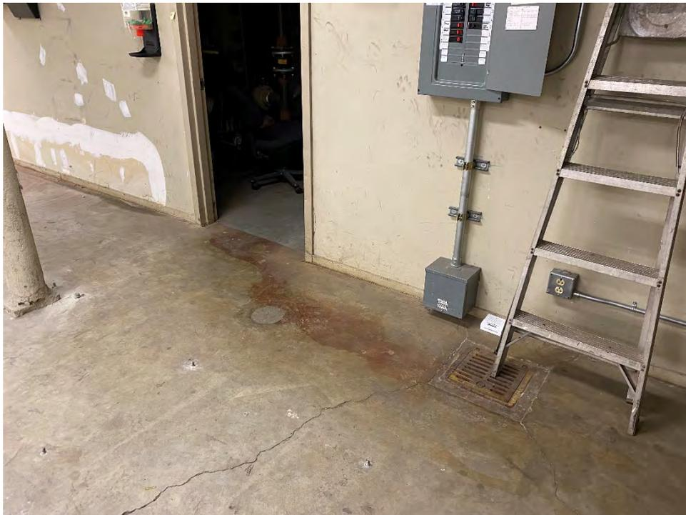
**Photo #8** View (facing southwest) of a rusted floor drain located adjacent to the basement stairs. Surficial staining was identified which appears to originate from the basement mechanical room.
