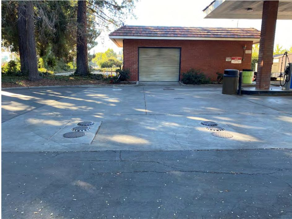
**Photo #23** View (facing south) of fill ports for two of at least three underground storage tanks associated with the fueling station located on the eastern-adjacent site. An unlabeled poly container is visible adjacent to the brick building.
