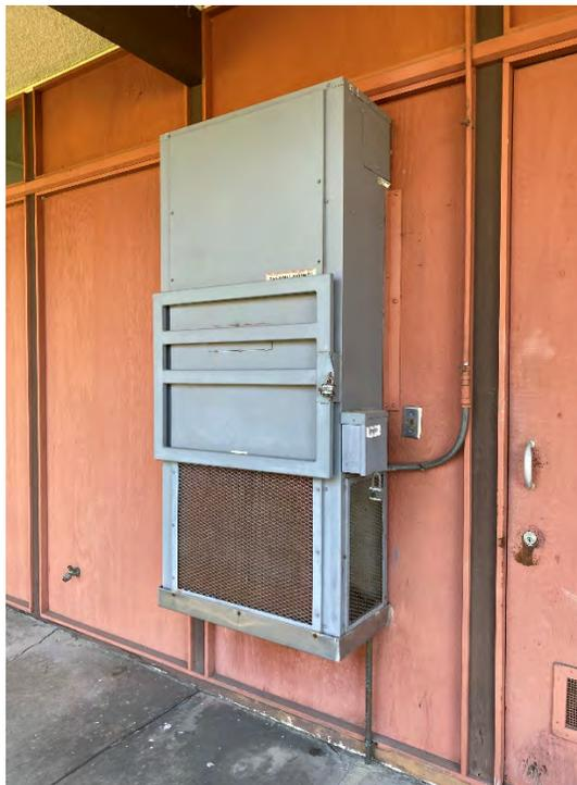
**Photo #16** View of one of four heat pumps located on the exterior of the Subject Property building (one at each of the four corners).
