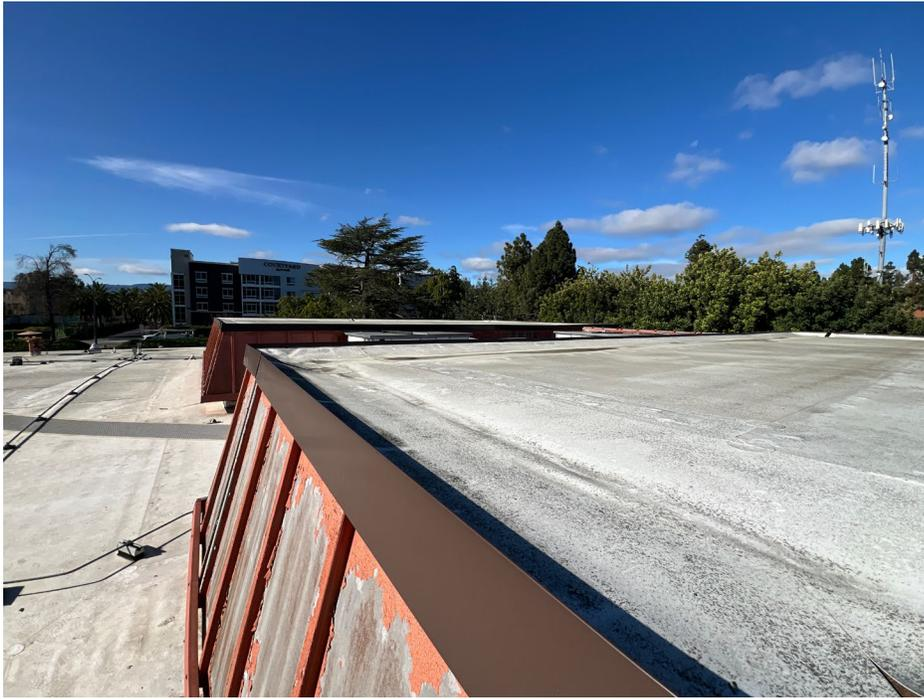
**Photo #11** View of the red paint (P01) on the Former Courthouse roof. This paint is lead-based paint (LBP).
