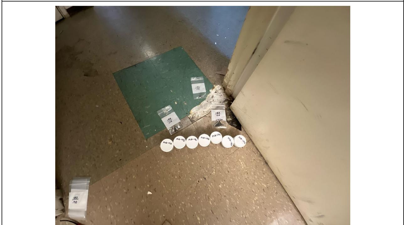
**Photo #6** View of tan/brown/green floor tile. The floor tile (HA #18) and associated black adhesive (HA #19) are asbestos-containing.
