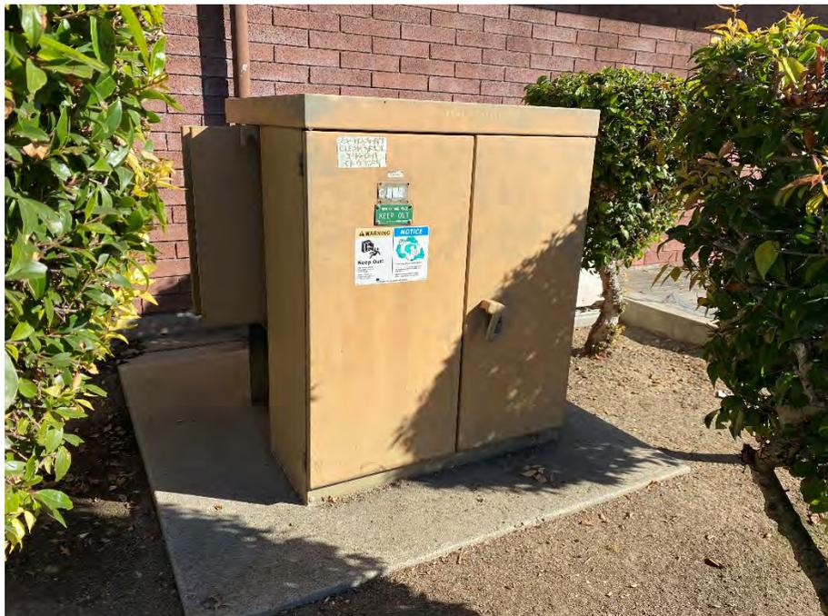
**Photo #18** View (facing northeast) of pad-mounted transformer located on south side of the building exterior.
