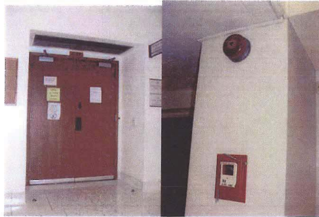
Fig. 9: Typical courtroom entry doors are too narrow and do not meet fire code. Courthouse lacks fire sprinkler and fire alarm systems.
