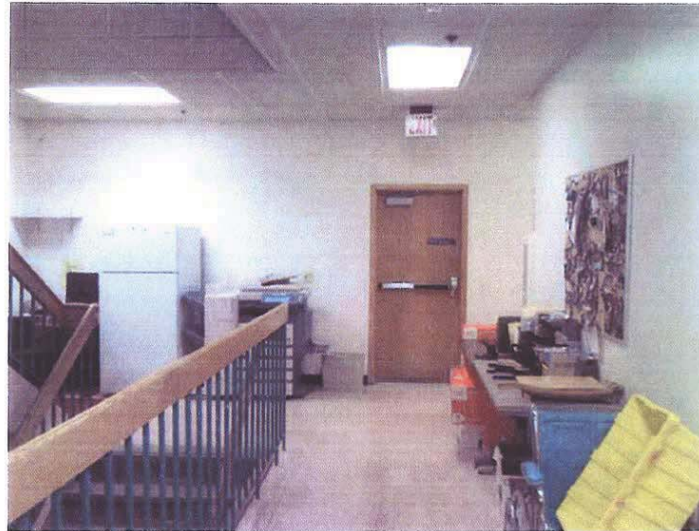
Fig. 17: Family Courthouse: Exit corridor is used for copy machine, storage and break area due to space shortage.
