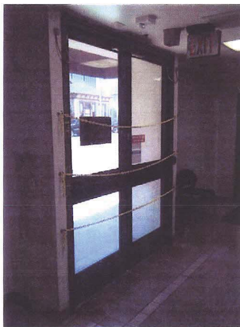
Fig. 16: Family Courthouse: Unsupervised exterior glass doors in public lobby pose perimeter security and exiting concerns.
