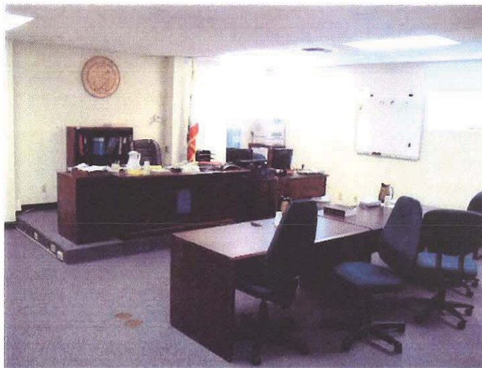
Fig. 24: Substandard Trailer C2 courtroom -- Desk for Judge's bench, no ramp or rail, limited public seating. Windows facing public parking lot create security risk.
