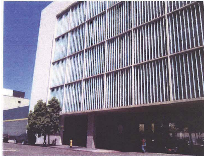
Fig. 2: Seismic fault lies beneath courthouse north tower
