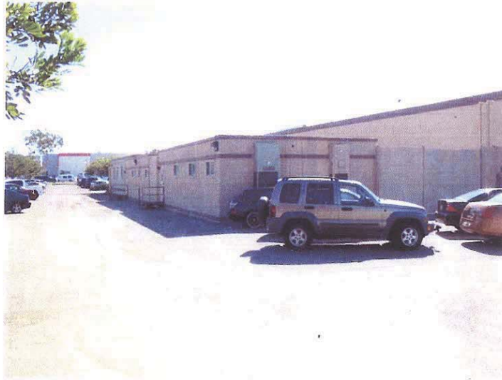
Fig. 23: Trailer C-2 backs up to public-accessible parking lot.
