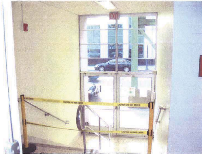
Fig. 12: Emergency exits are blocked off due to security concerns. This photo also illustrates ADA and fire exiting issues.
