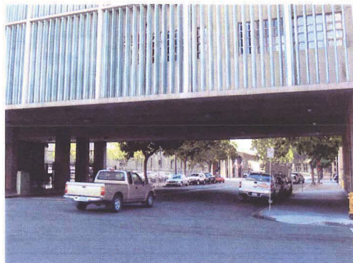
Fig. 3: Courtrooms and chambers span over two city streets. Shown above is building spanning B Street as viewed from the corner of "B" and Union Streets.
