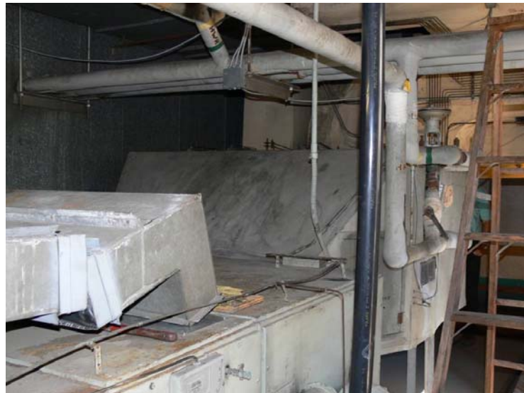
Fig. 11: Original air-handlers from 1961 have long exceeded their useful life.
