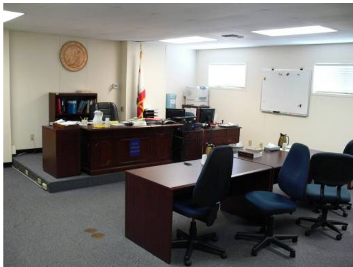
Fig. 24: Substandard Trailer C2 courtroom -- Desk for Judge's bench, no ramp or rail, limited public seating. Windows facing public parking lot create security risk.
