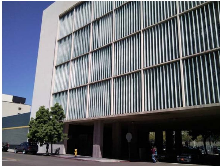
Fig. 2: Seismic fault lies beneath courthouse north tower
