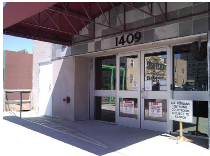
Fig. 21: Madge Bradley: Lack of back up vertical transportation forces the use of an unsecure fire stair (white door at left) when the only public elevator breaks down.
