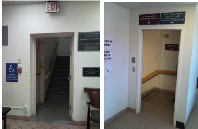
Fig. 15: Family Courthouse: Inaccessible ADA public path (actually fire exit stairs) from courtrooms to family services offices. Public must go up and down two flights of stairs to get to the business office, children's waiting room and Family Court Services due to awkward addition to building.
