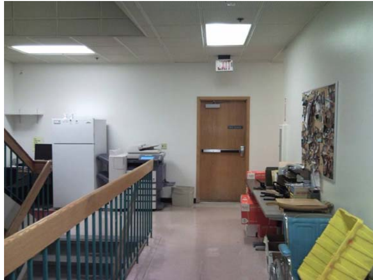
Fig. 17: Family Courthouse: Exit corridor is used for copy machine, storage and break area due to space shortage.
