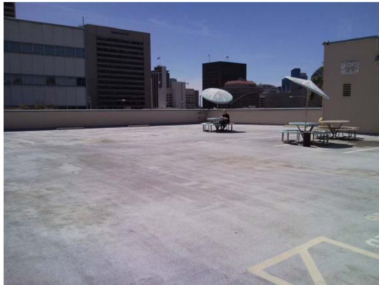
Fig. 19: Family Courthouse: Rooftop parking has been abandoned due to structural deficiencies.
