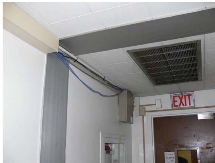
Fig. 10: Due to presence of asbestos above the ceiling throughout the courthouse, cables and conduit are installed below the ceiling, including in exit corridors as shown.
