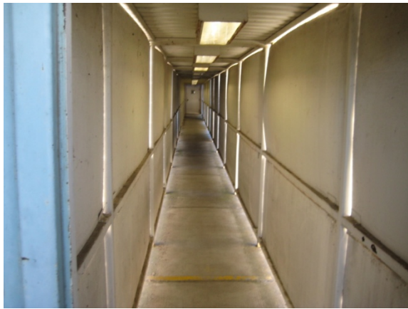
Figure 17. Elevated inmate walkway through holding to courthouse
