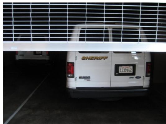
Figure 6. Sally port entrance
