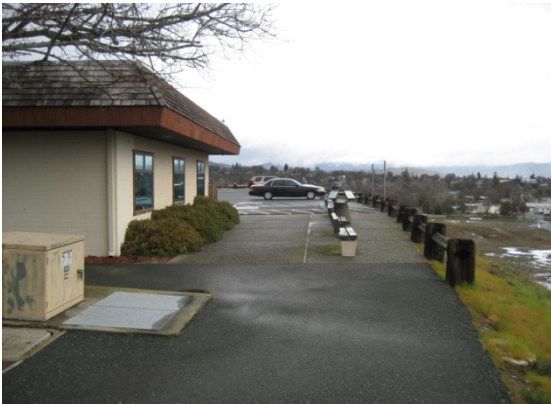
Figure 4. The Chamber of Commerce building and adjacent parking area
