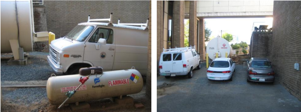
Photos of the two fuel tanks located between the courthouse on the left and the old jail on the right.
