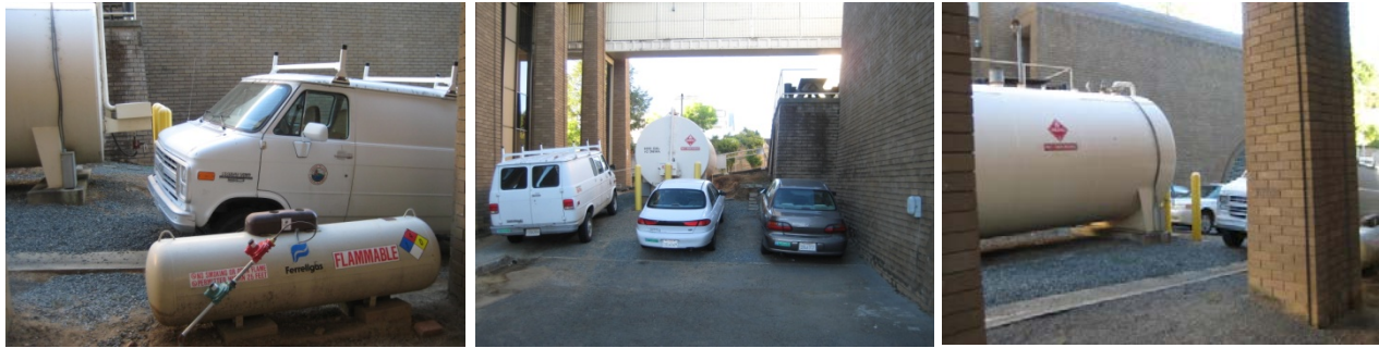
Figures 7–9. Diesel and propane storage between buildings
