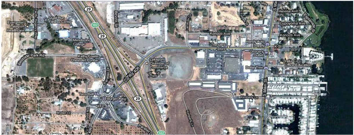
Figure 1. The Lakeport Boulevard building site. The court will be located on in the flat open area just right of the Chamber of Commerce. Lakeport Boulevard is the road directly above the site.
