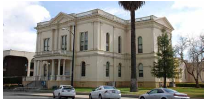
Current image of Courthouse from Northwest.
